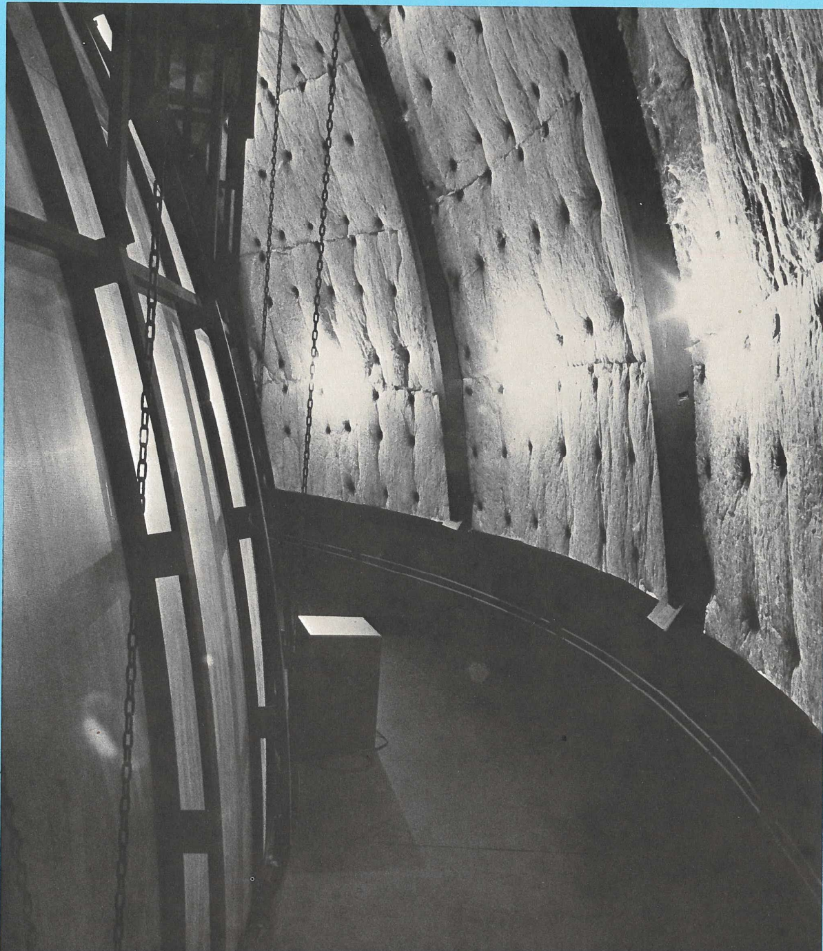
The fifty-foot perforated aluminum inner dome is entirely suspended from the larger outer dome. The five-foot catwalk space between the domes provides space for the speakers of the Omniphonic sound system, for air-conditioning, and for various special effects.
