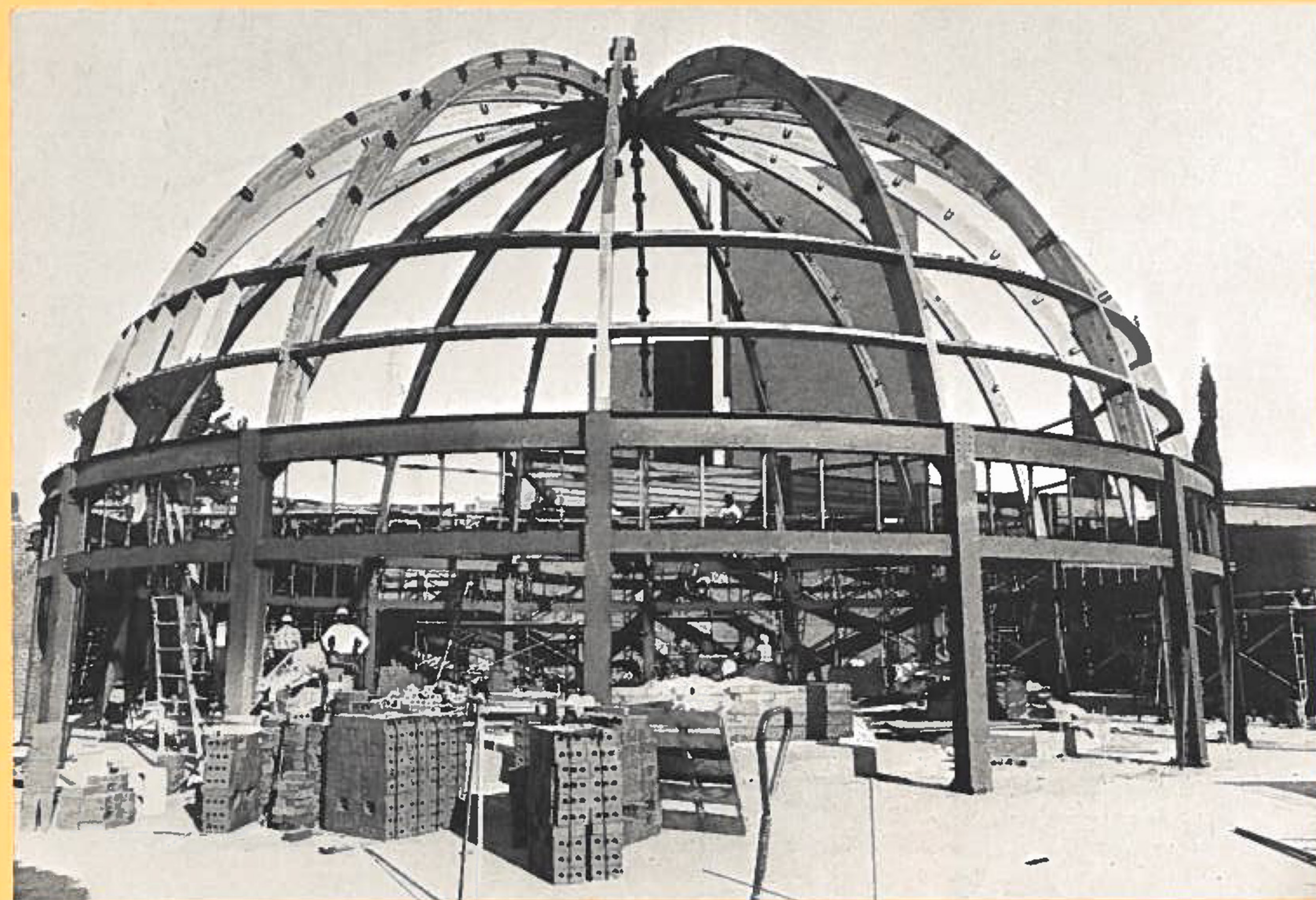
March 1975: Laminated wooden beams form the Theater dome.
